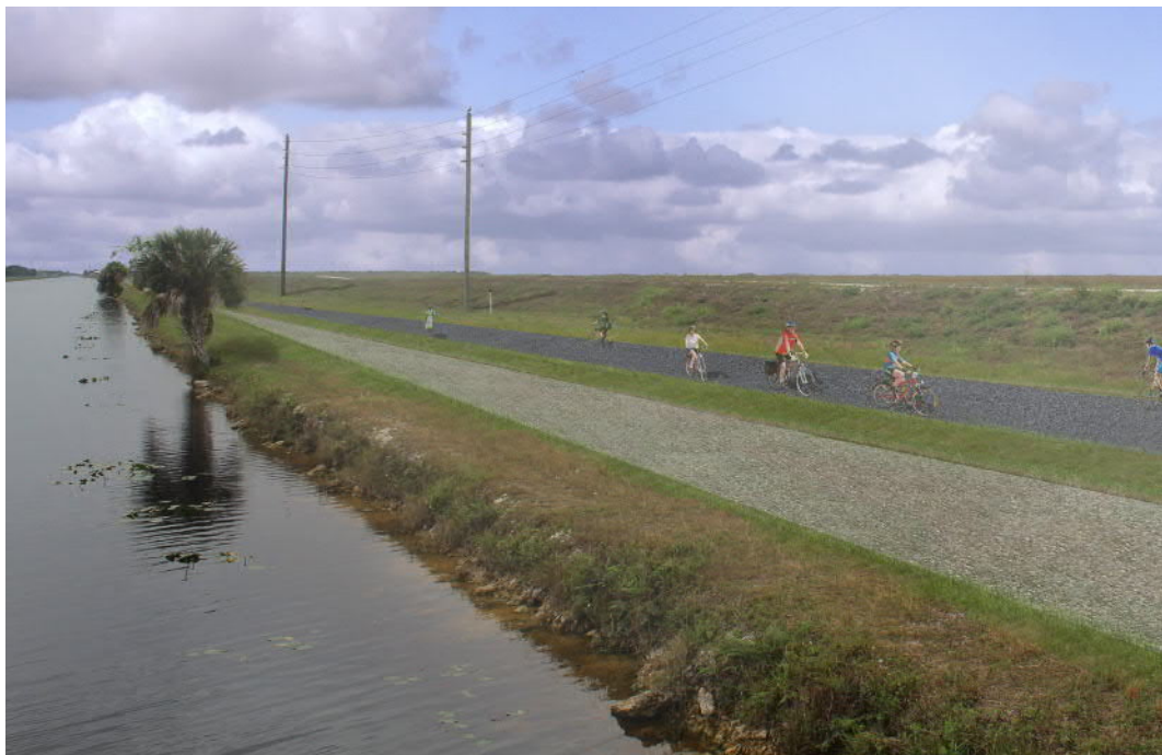
03 Path on Levee Bench (L-29 Levee - ROGG East) (within SFWMD right-of-way)
